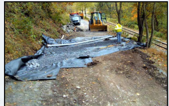
Installation of French Mattress
