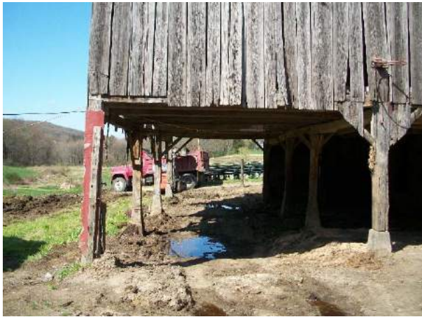
Wade Fisher Farm – Former heavy use area.
