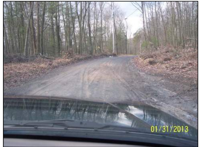
Road ruts and poor drainage
