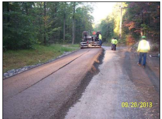
DSA placement in 6" or 8" lift. See shoulder stabilization on left.
