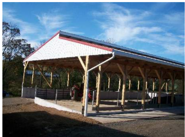
Rob Witmer Farm – Concrete and gravel heavy use area, as well as gutters.
