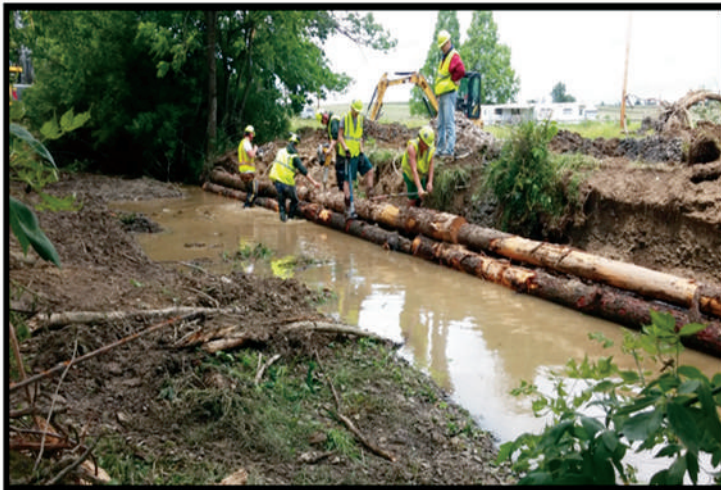
2016 Stream Restoration project. Partners- NPC, PA DEP, PA F&B, local landowners, youth volunteers.
