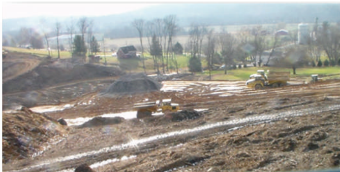
View of earthwork from a point east of SR 147 looking west toward the Robert Snyder Farm, which is located west of SR 147 and south of SR 405.
