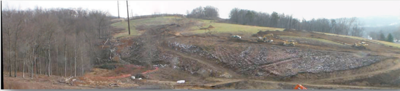
Area southeast of intersection of SR 405 with SR 147 being prepared for stream relocation under thruway via 66' culvert.
