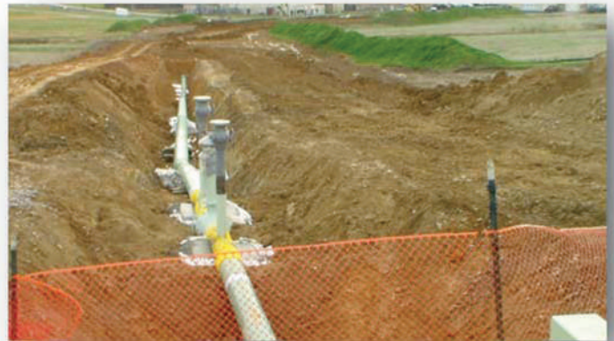
A mainline valve has been installed in the pipeline south of Ridge Road. This portion of trench will be backfilled after surface restoration plans have been approved and implemented.
