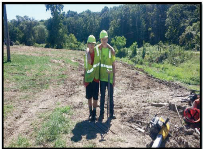
2016 Stream Restoration project. Partners- NPC, PA DEP, PA F&B, local landowners, youth volunteers.
