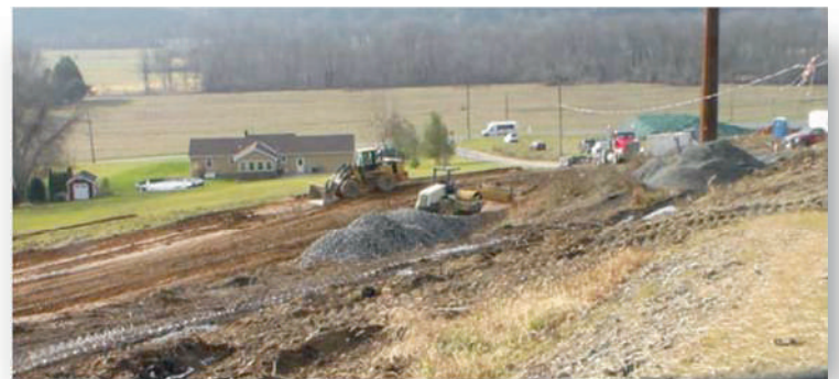
View of earthwork in the vicinity of Acorn Drive looking at the intersection of Acorn Drive with SR 147 .
