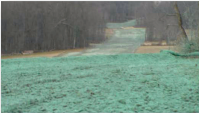
Pipe line has been installed and the trench backfilled, topsoil replaced on the right-of-way and stabilized with seed and mulch.
