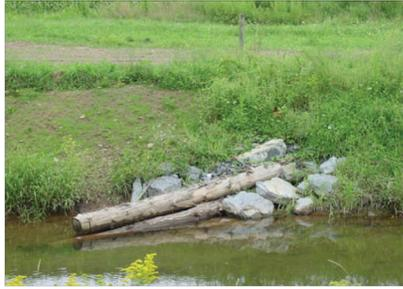
A combination of 10 multi-log vane deflectors, two singles log deflectors, stream bank fencing and a stream crossing were installed through a Chesapeake Bay Mini Grant on the Mahantango Creek in the summer of 2009. The log deflectors redirect the flow of the stream to the center of the channel, reducing erosion while creating habitat for aquatic species.
