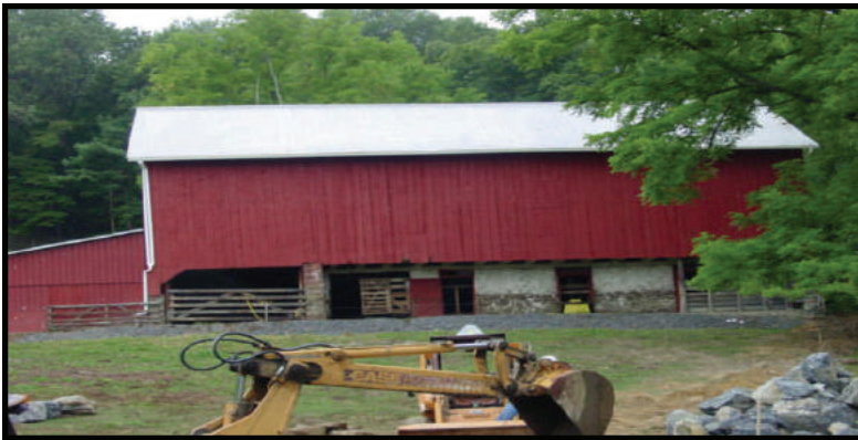
This is a roofed structure built to control runoff from a beef cattle feedlot.
