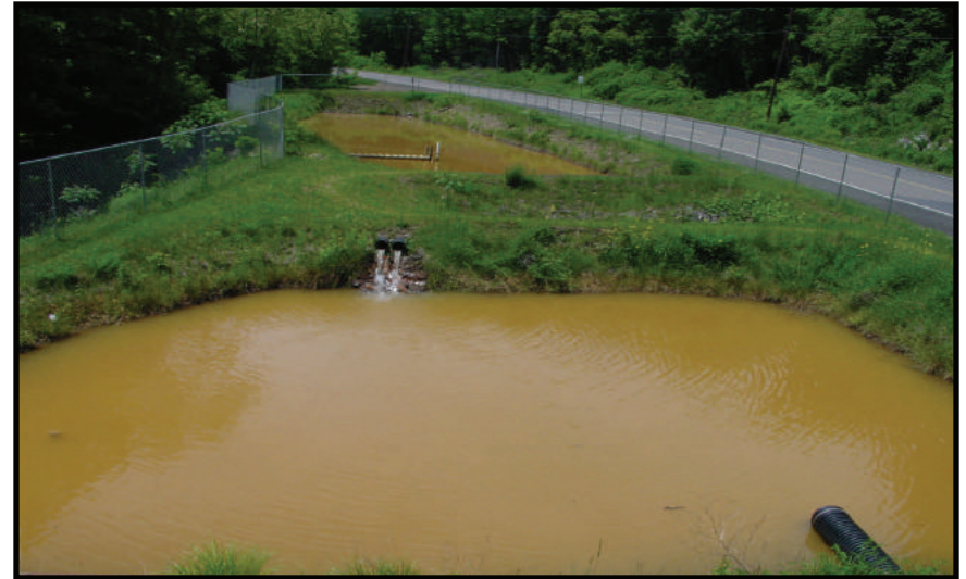
The top photo shows one of the various Acid Mine Drainage treatment systems installed in Northumberland County. This system is located in the Shamokin Creek Watershed and is designed to treat the polluted water discharge before it enters the main stem of the Shamokin Creek. The photo below shows the installation of a vegetative buffer along a stream bank in the Little Shamokin Creek watershed, where plant roots will absorb excess nutrients and hold soils in place.
