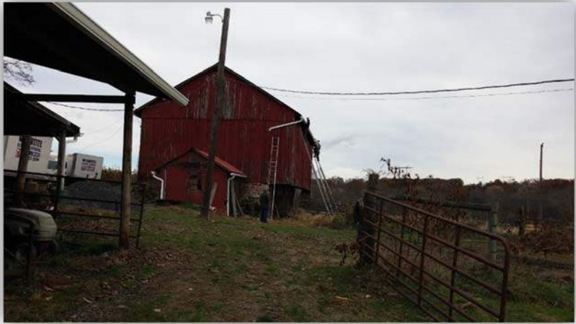
Adding gutters and downspouts to the Reader barn- keeping clean water clean
