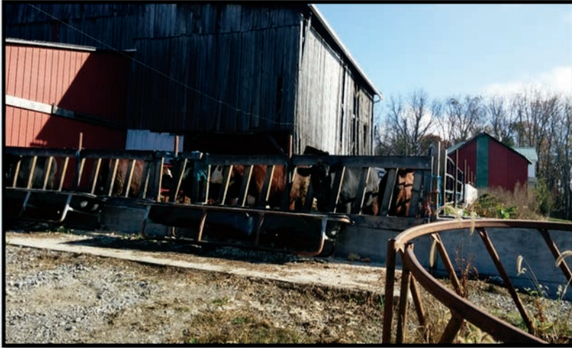
Fisher barnyard after project construction
