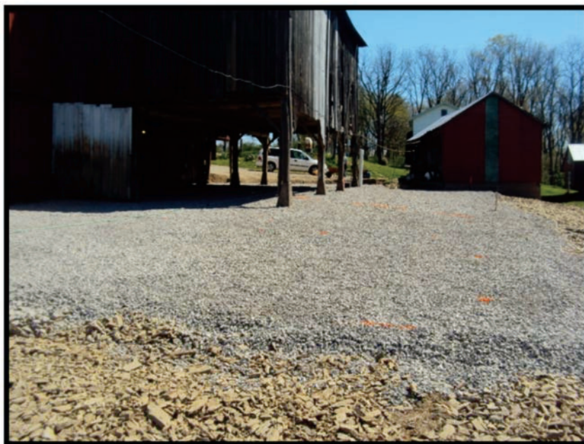
Fisher barnyard during project construction
