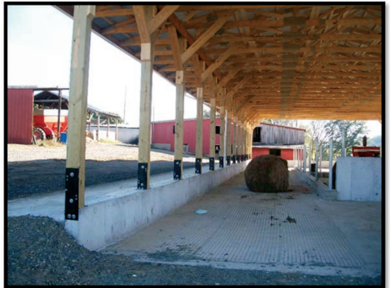
Witmer barnyard during project construction
