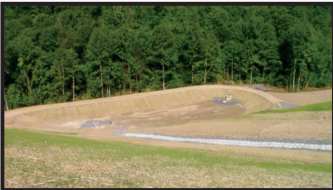
Stormwater Basin and Diversion Swale
