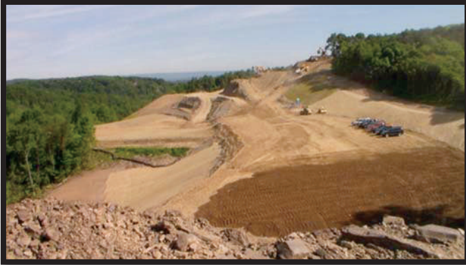
Earthwork for Southern Approach
