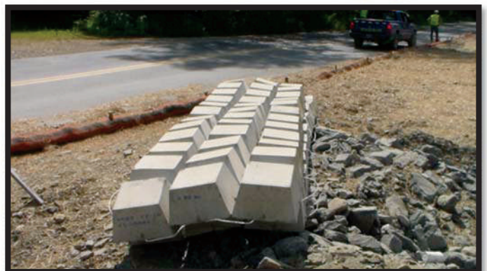
Section of Concrete Revetment
