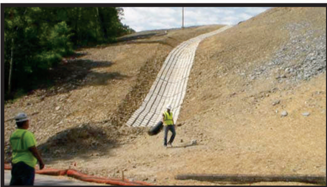
Drainage Swale with Concrete Revetment
