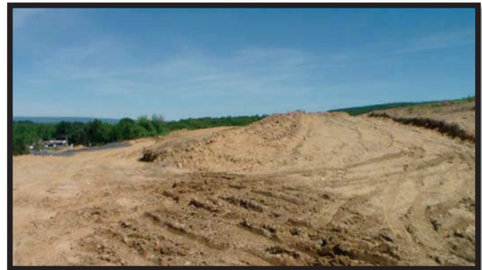
Earthwork for Northern Approach
