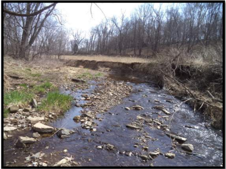
Before: Unstable, vertical banks along outside of meander
