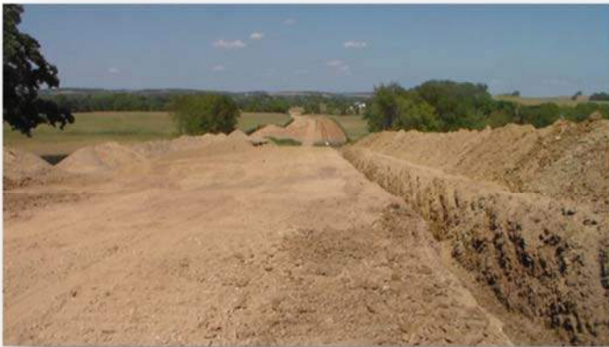
Right-of-Way with topsoil stripped and stockpiled along the side
