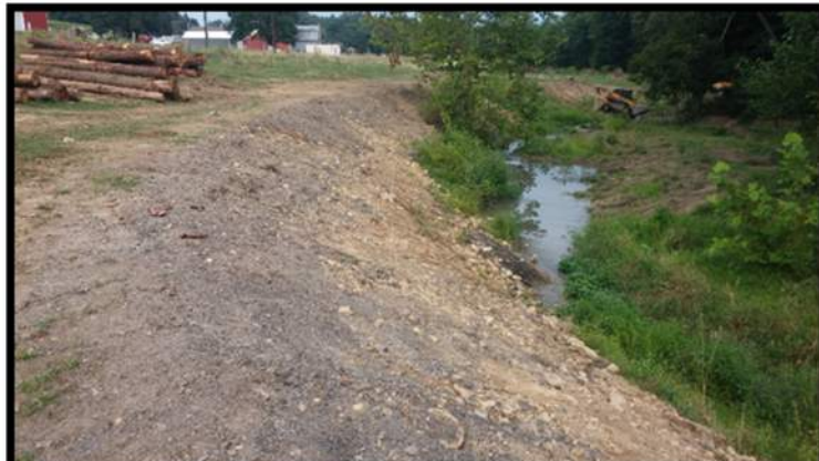
After: Graded, stabilized streambank on outside of meander
