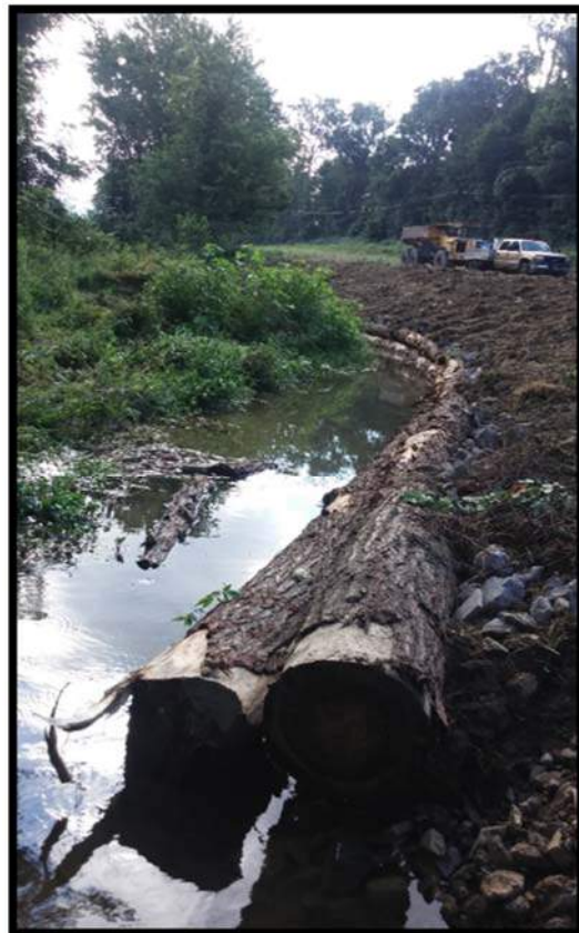
After: A modified mudsill with regraded banks stabilize this long, outside meander
