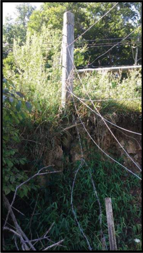
Corner fence post was about to fall into stream channel
