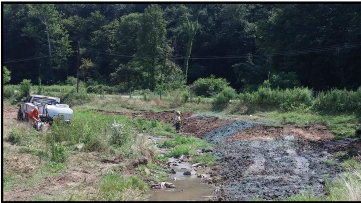
All bare soil areas were covered with hydro seed
