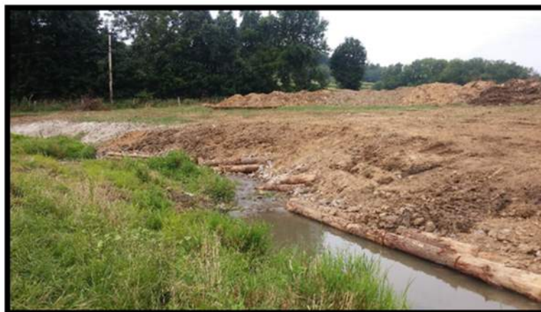
After: Multi-log deflectors and toe logs protect streambank
