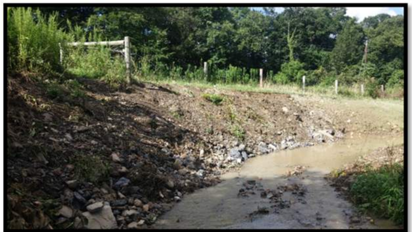
After: Vertical bank was regraded to reduce erosion at toe of bank and restore functionality during high waters
