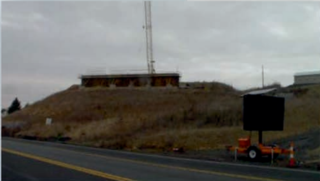
Abutment construction as viewed from SR 0147
