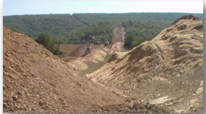
Right-of-way after pipe was installed, trench backfilled and seed and mulch was applied. From Snyder Road looking South over Montour Ridge in East Chillisquaque Township.
