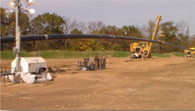
Welded pipe being fed into boring under Susquehanna River in Point Township.
