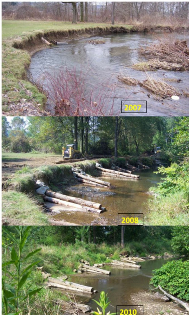
Figure 2: Stream bank erosion stabilization time lapse using multi-log structures. These structures are dual purpose in providing aquatic habitat and water deflectors to reduce stress on the banks.
