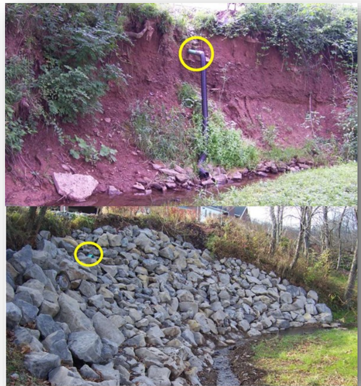
Figure 3: Stream bank erosion structure with rip rap offers bank stability.
